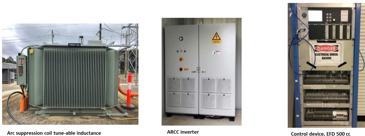
Figure 5: Three components to ARCC technology
