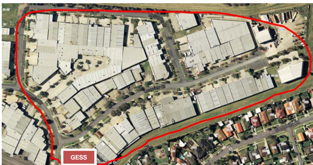
Fig 4: Aerial view of the customers that can be supplied solely by the GESS in 'island mode'
