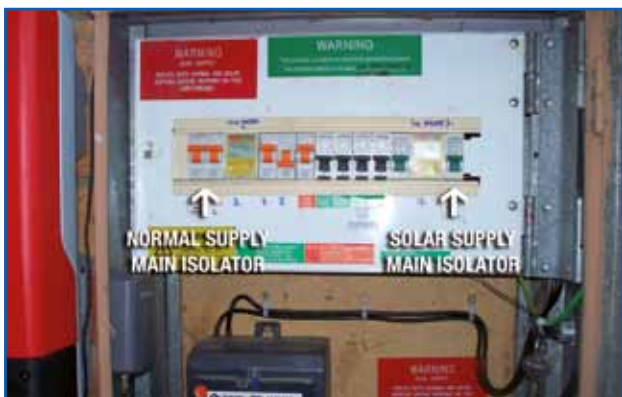
Figure 1 – Powerboard
